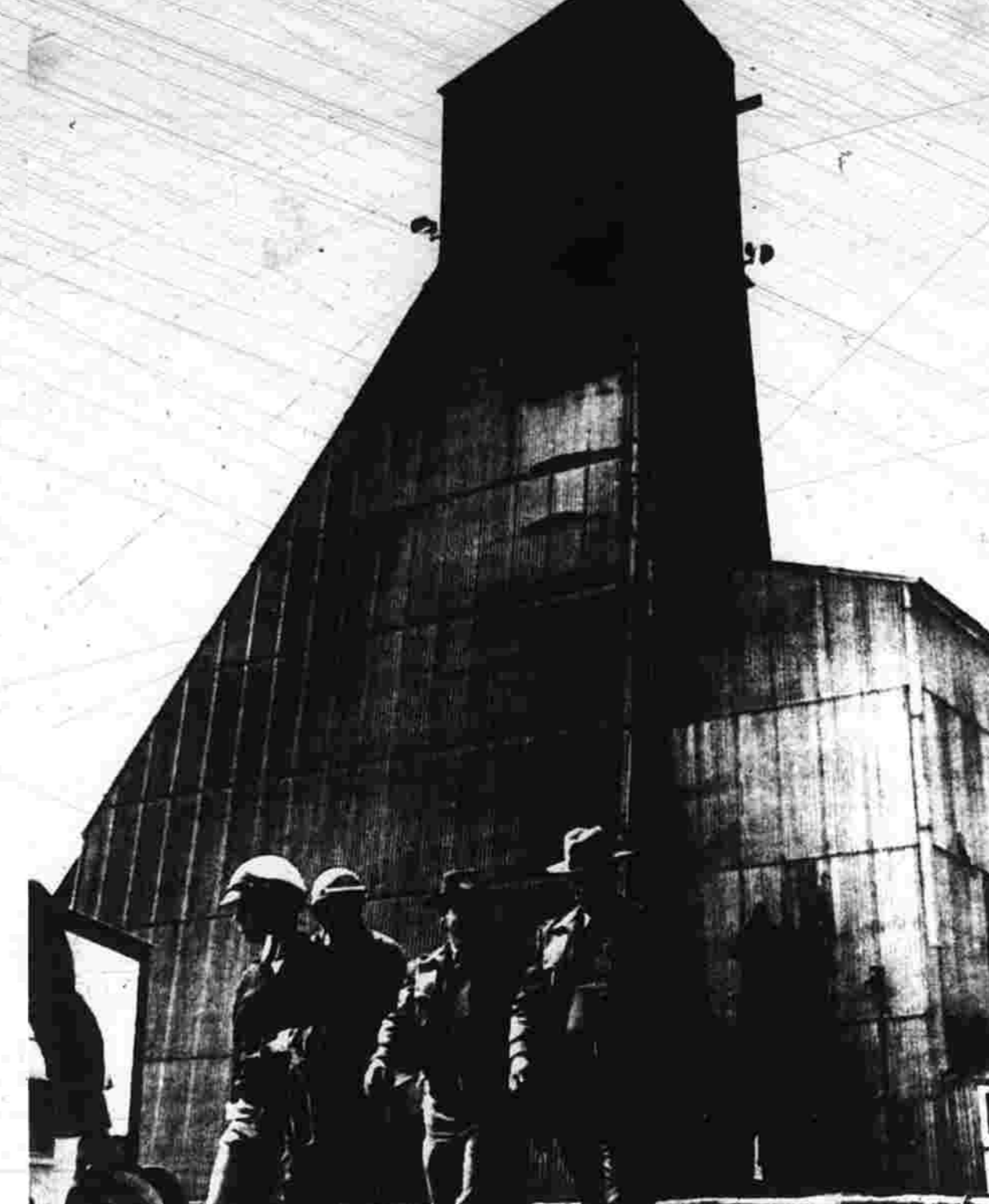
Shaft where 21 miners were trapped in Calumet, La. (AP Photos)
